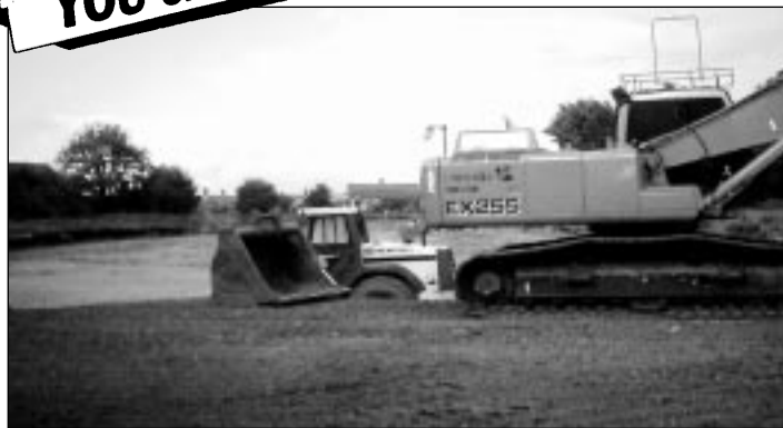
SKF site on the High Street
